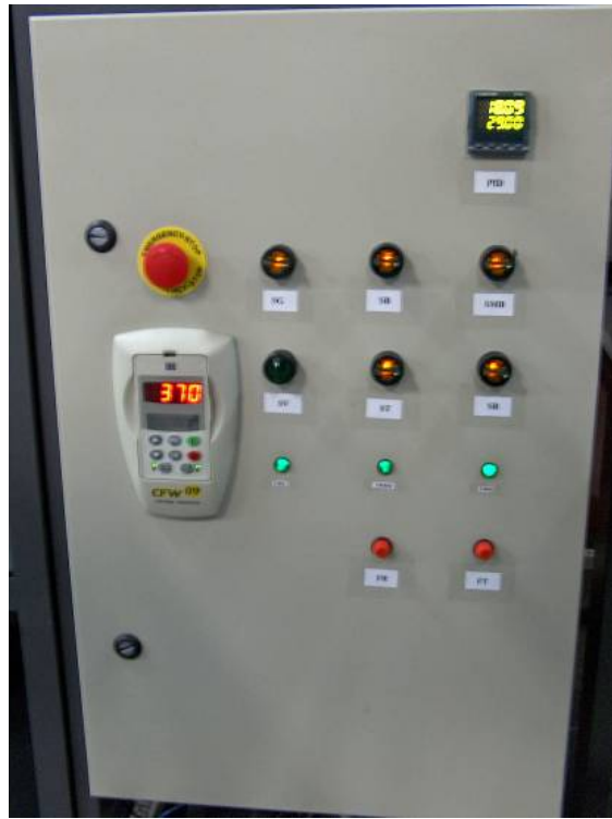
Figura 3.23 – Painel de Controle.
